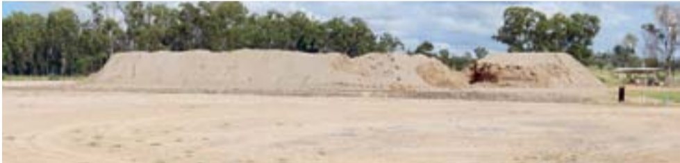
Concrete on site has been recycled into road base material.
