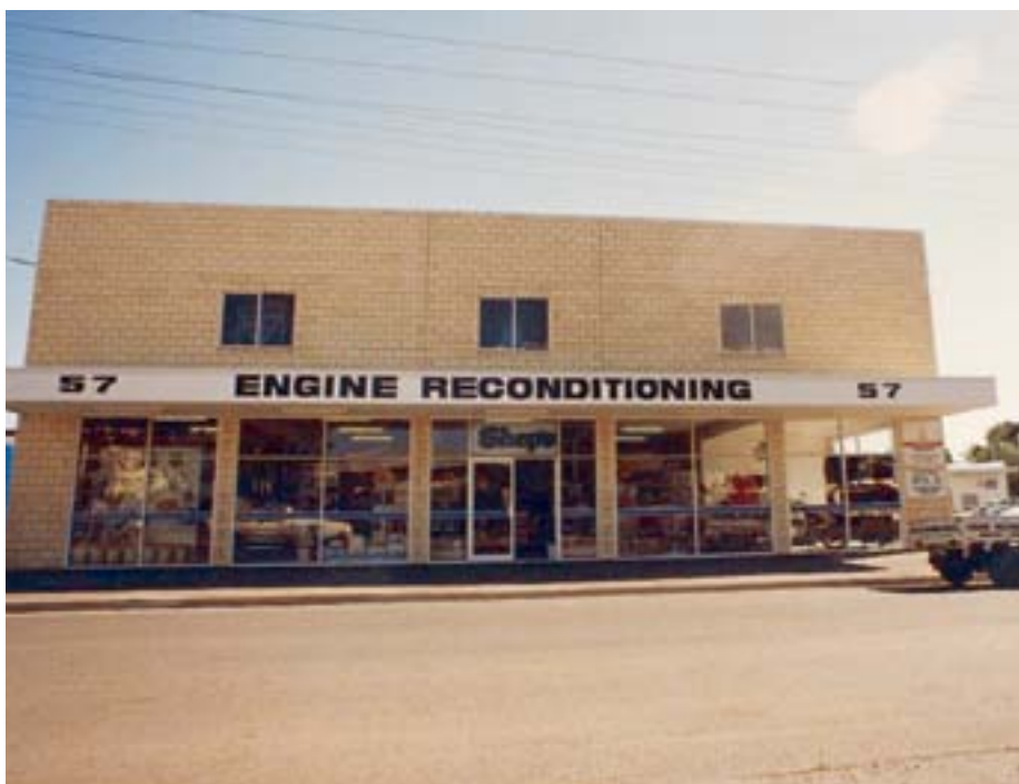
The latest workshop, front view.
