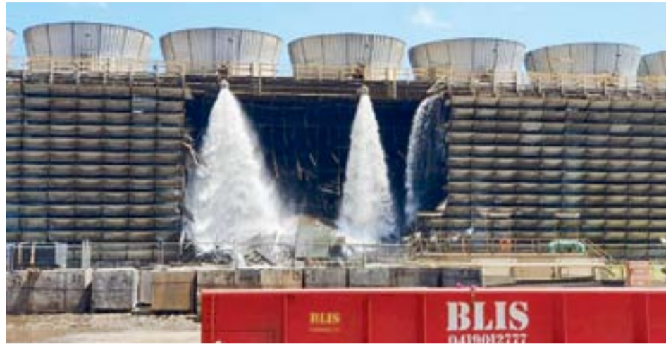
Return to service dates for Callide C Power Station units C3 and C4 have been delayed until 2024. Picture: SUPPLIED
