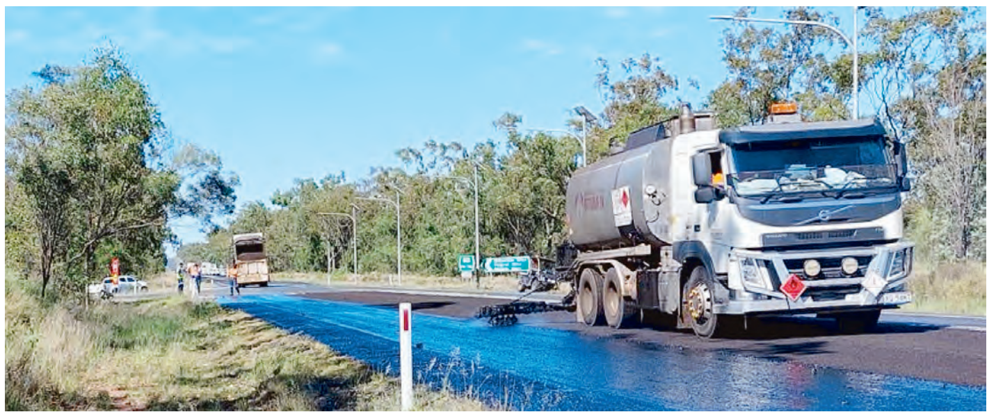
For the first time in Queensland, mining tyres were used to seal the roads.
