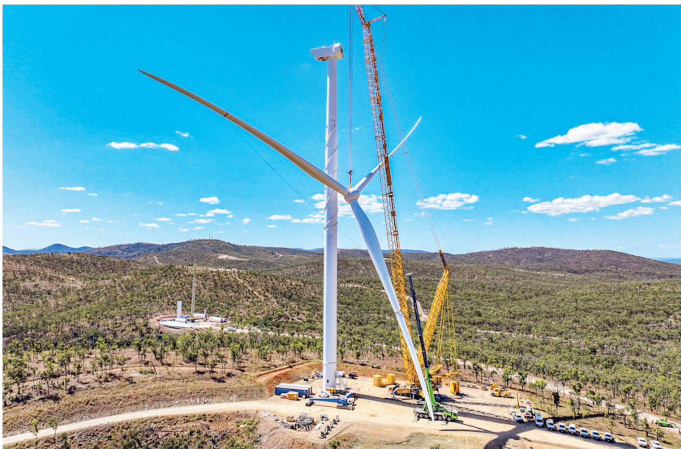
The first turbine in Clarke Creek has been built.
