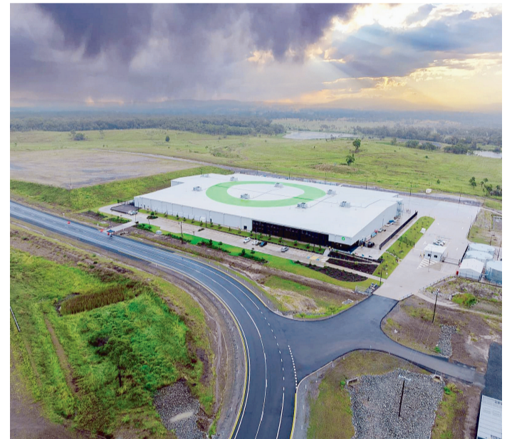
Fortescue's new Electrolyser Facility at Aldoga. Picture: DEPARTMENT OF THE PREMIER AND CABINET
