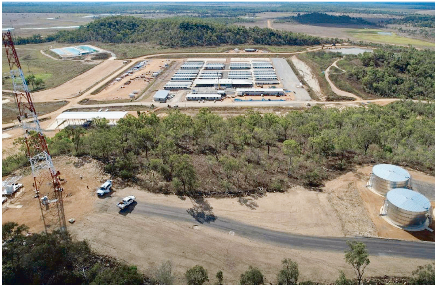
An aerial view of the $1 billion Australian Singapore Military Training Initiative project at the Shoalwater Bay Training Area.
