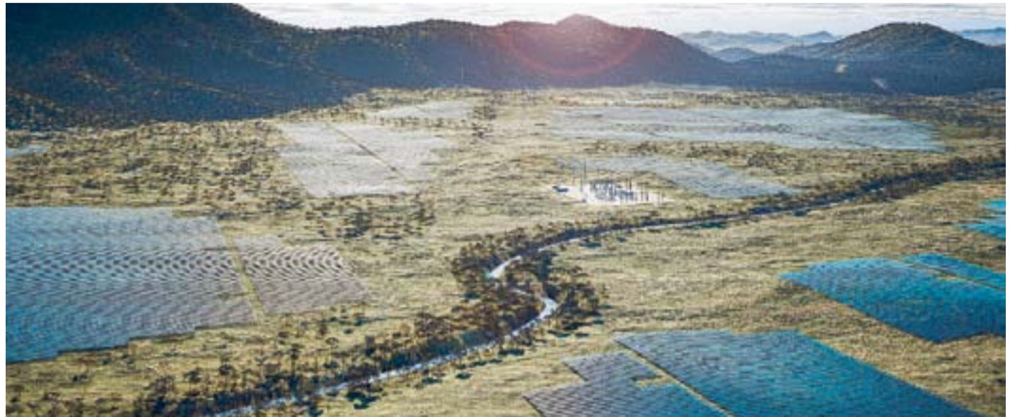
Renewable energy takes centre stage in Central Queensland with Acciona Energia's Aldoga Solar Farm near Gladstone.
