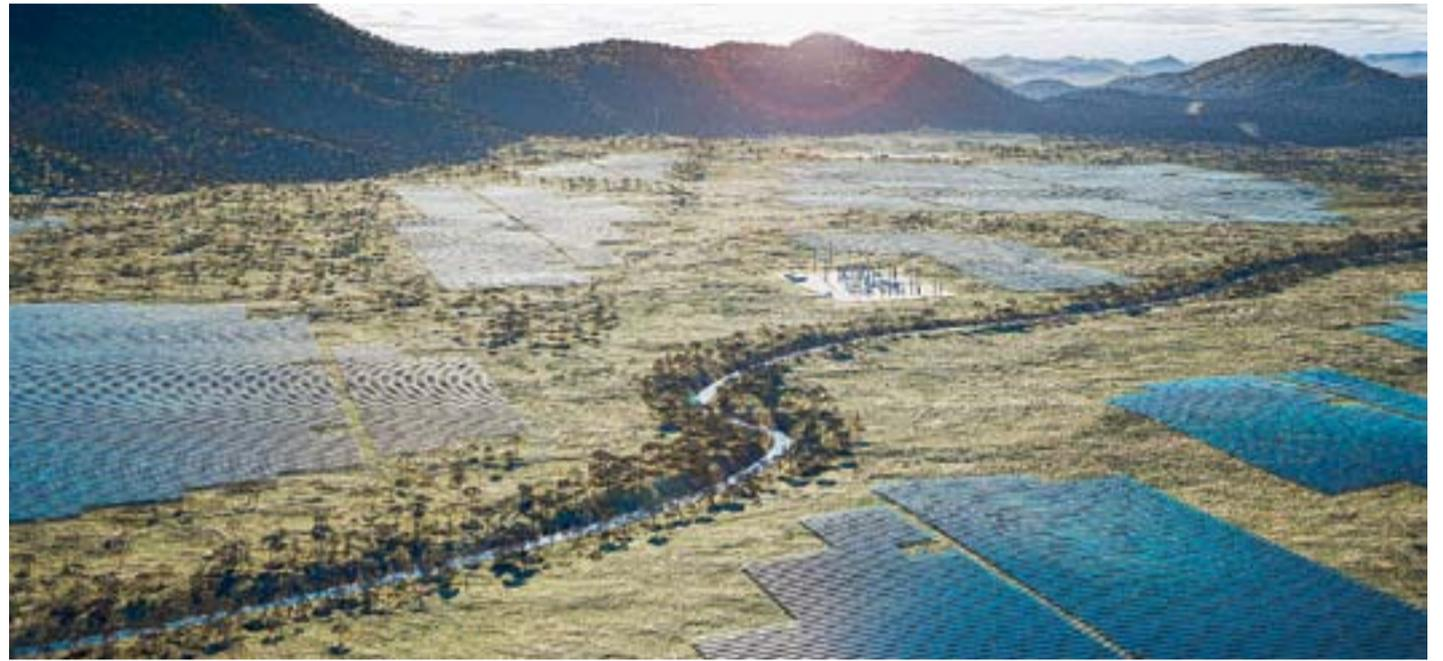
The \$500 million Aldoga Solar Farm will feature up to 820,000 solar modules with the capacity to produce 480 megawatts at its peak.
